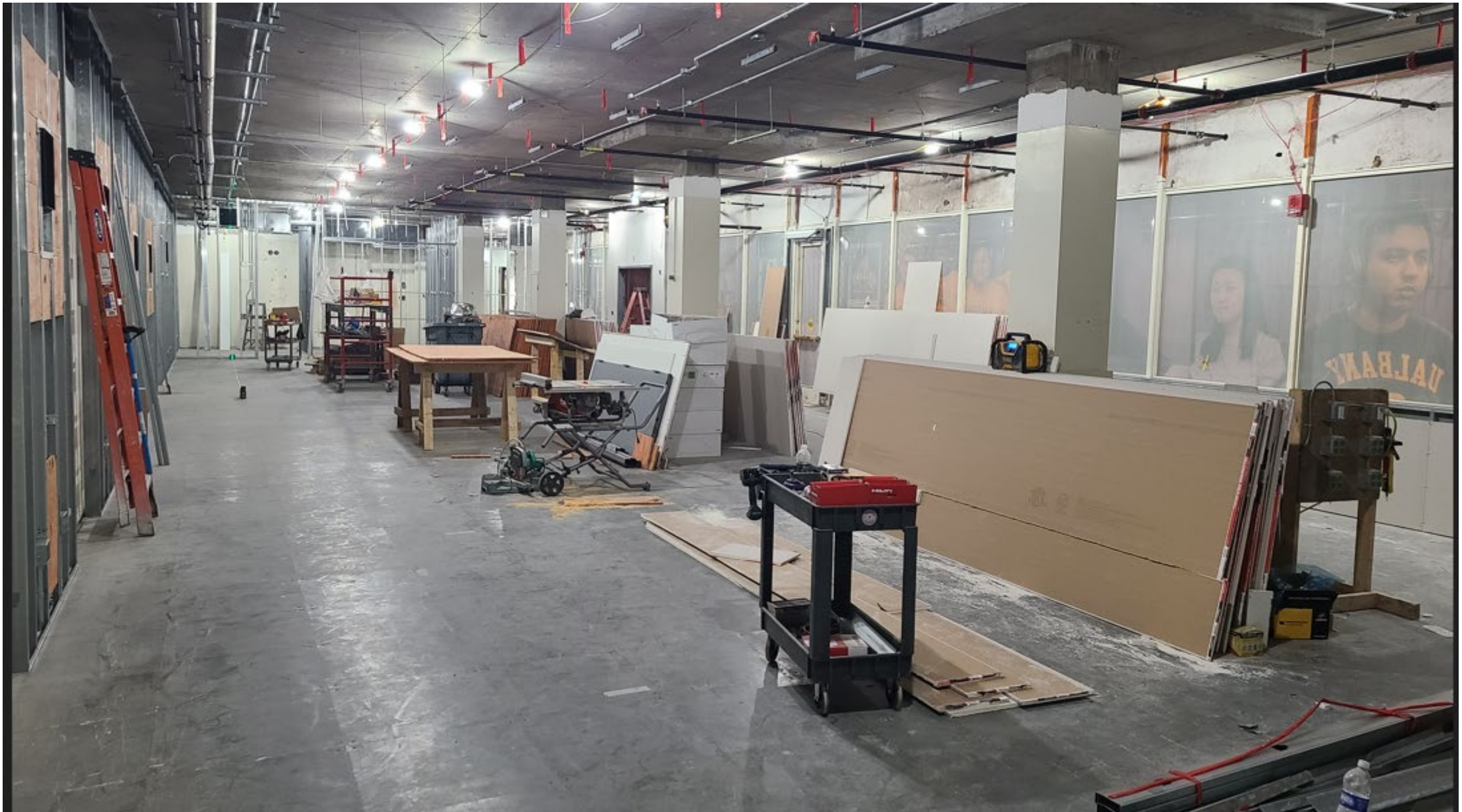
Current Photo – Under Construction
