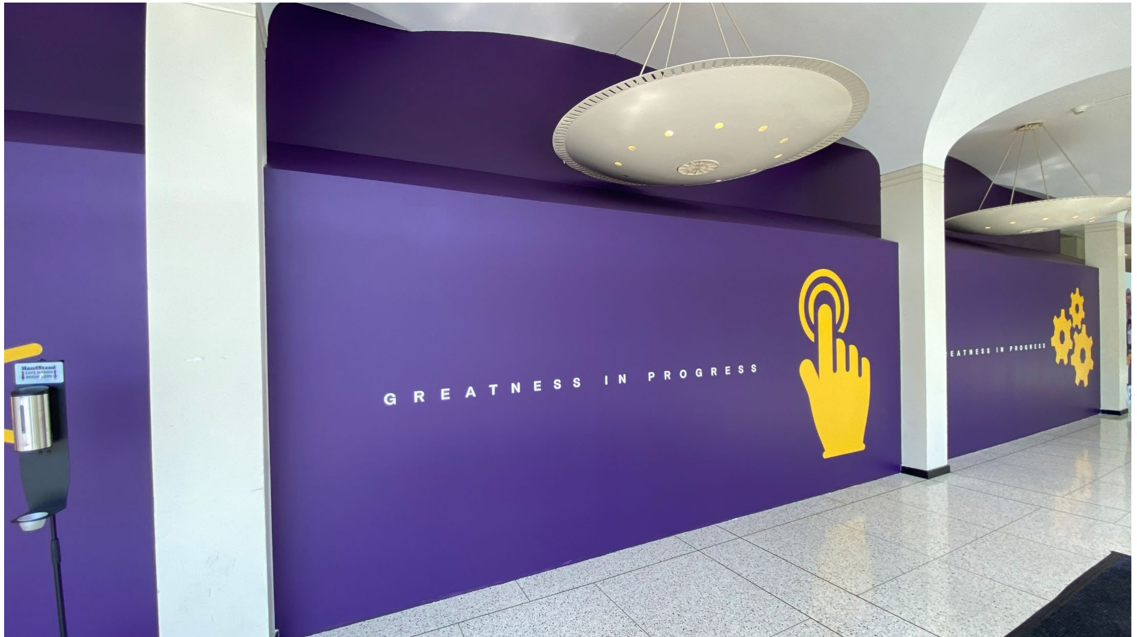
Temporary Enclosure During Construction – Minimize Disruption
