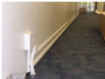
Surface mounted wiring in the Library, basement reading room
