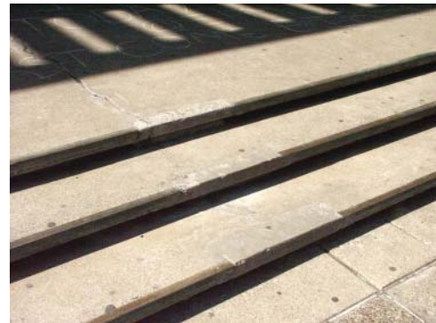
Cracked and repaired stairs.
