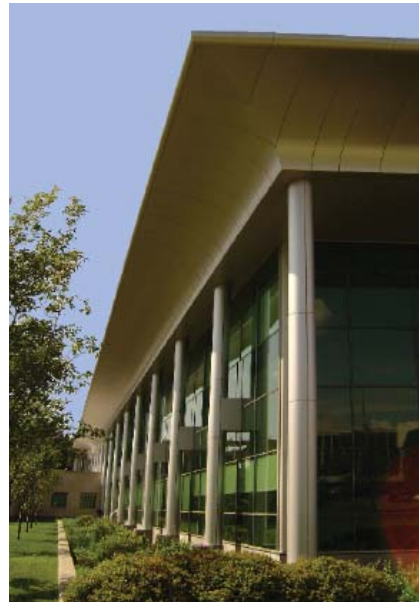
An updated version in silver aluminum formed panels on the Life Sciences Building.
