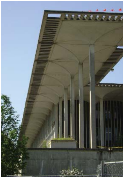
Stone's original pre-cast concrete overhangs on the Podium.
