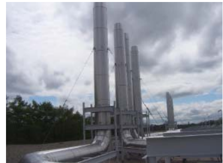
Fume hood exhaust ducts above the Chemistry Building
