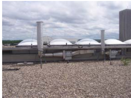
Fume hood exhaust ducts above the Earth Science Building
