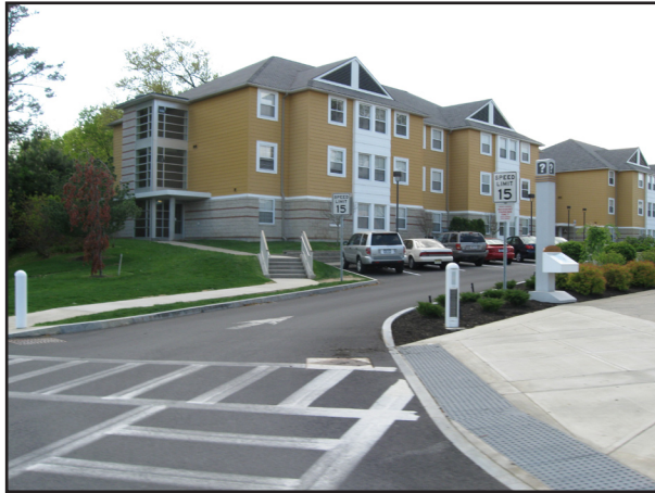
Fig. 33: Wide, Gentle Curb ramp at Empire Commons
