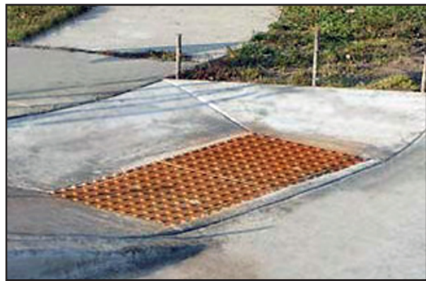
Fig. 34: Curb ramp with Cast Iron Detectable Warning: Oxidized iron provides the required contrast with adjacent pavement
