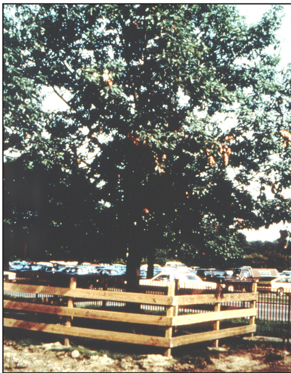
Fig. 52: A durable tree protection fence in use on a construction site
