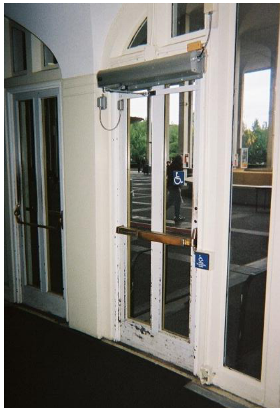
Door with Deteriorating Finish
