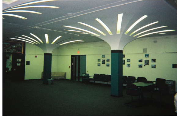
Lighting in Concrete Columns
