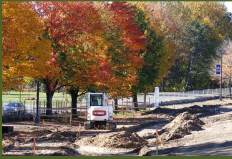
Construction of the Purple Path.
