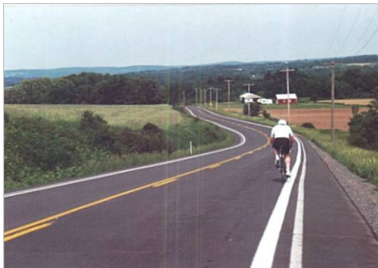
This road shoulder was widened, providing an improved facility for pedestrians, bicyclists and motorists.
