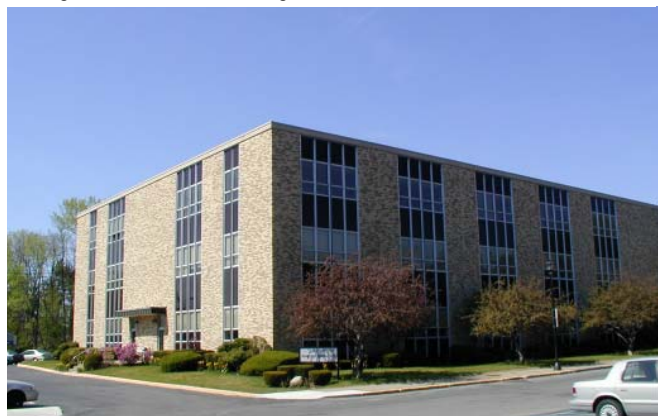
Management Services Building
