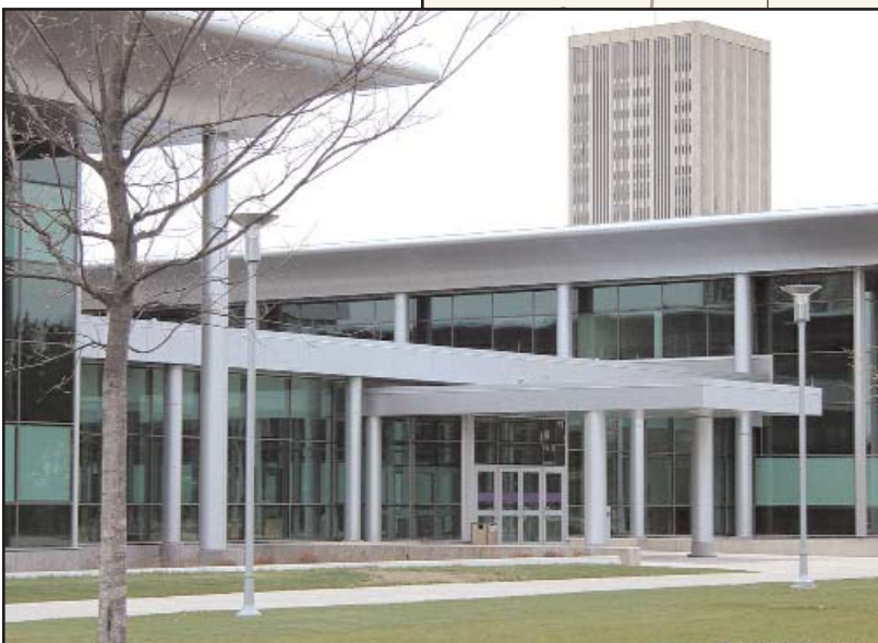
University at Albany Life Sciences Building
