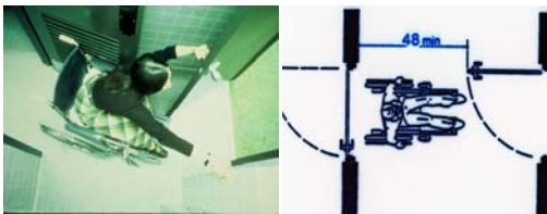
This woman is having difficulty getting through two doors positioned too close for maneuvering.
