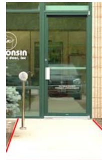
Figure illustrates maneuvering clearance at a swinging door.
