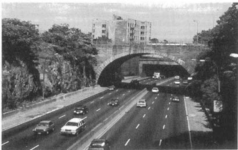
The Cross-Bronx Expressway trench through East Tremont in Summer 1991. View is looking east from Arthur Avenue
