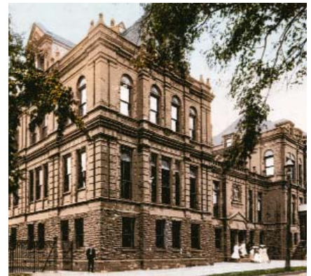
The Willett Street building
